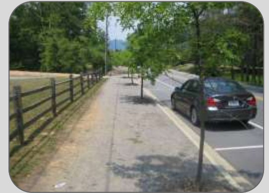
E: Gravel sidewalk along the NC Highway 9 near Black Mountain, NC.
