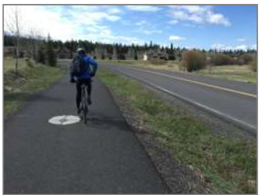
The sidepath recommended along Lovelady Road is a common treatment for multi-use trails. The example above has a drainage swale between the roadway and pathway.
