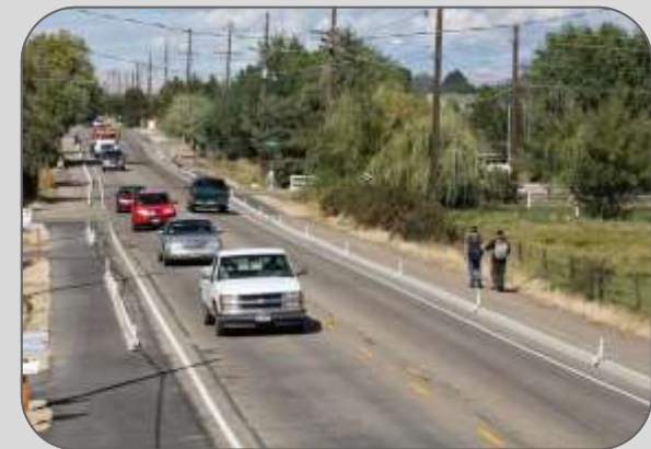
F: Shoulder/extruded curb pathway in Ada County, Idaho (constructed with federal Safe Routes to School funds)
