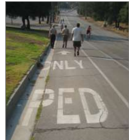
Excessive road width offers an opportunity for non-traditional (and less expensive) facilities. An option like shown above, with some type of vertical curbing between the walkway and travel lanes could be explored.
