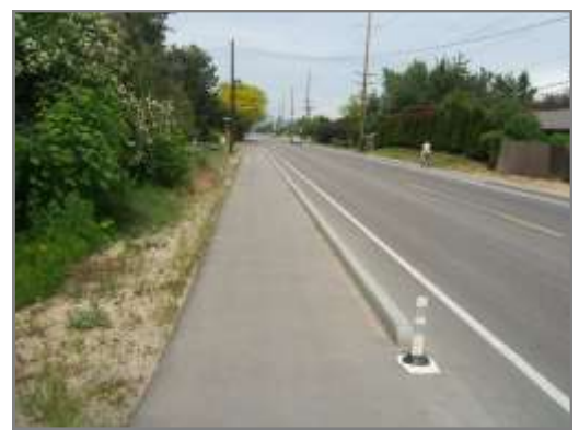
Non-traditional sidewalks, such as an extruded curb treatment (shown above), can be as effective as sidewalks while providing a lower cost option stretch limited funds while addressing basic needs.
