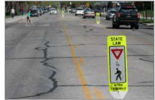
Pedestrian crossing panels can be placed at legal marked crosswalks at unsignalized intersections or other crossings to alert motorists of their responsibility to yield to those who walk.
